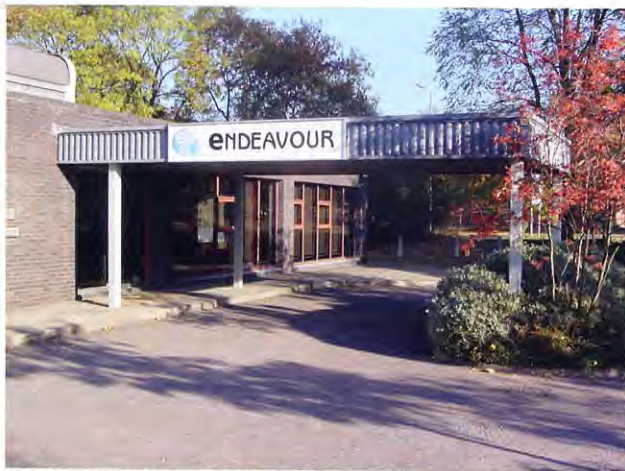
Endeavour Speciality Chemicals' Daventry, UK, headquarters.
